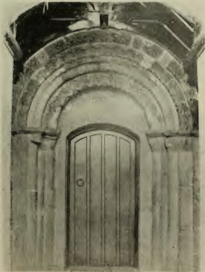
PLATE CIX. St. Martins-by-Looe. North Doorway
